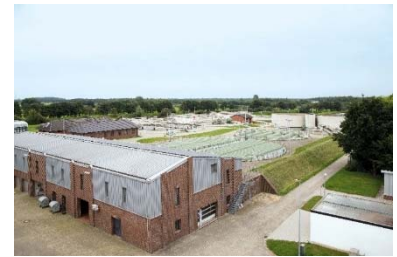
Edeweicht wastewater treatment plant
