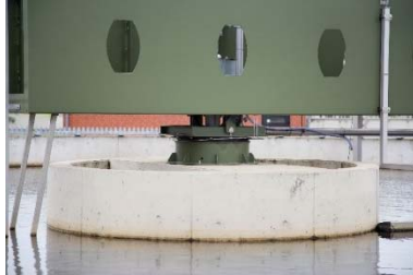
Central slewing ring with automated lubrication technology
