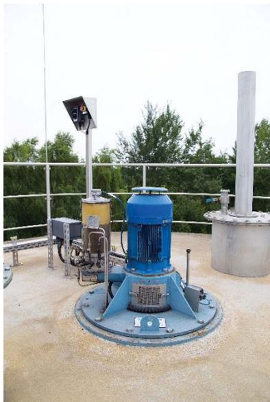
Stirrer digestion tower with central lubrication
