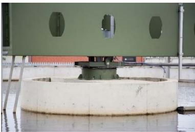
Central slewing ring with automated lubrication technology
